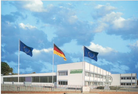
Production plant in Neuenhaus
